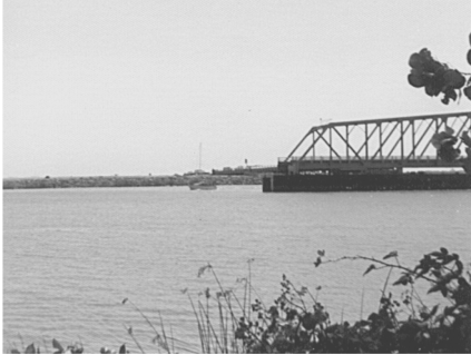
Mokelumne River Swing Bridge
