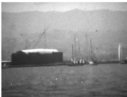
Howard Hughes Mining Barge HMB-1
