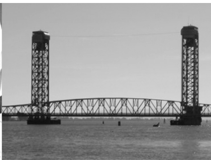
Rio Vista Bridge
