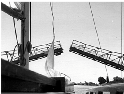
Isleton Bascule Bridge
