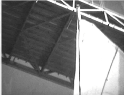
Passing under Oakland Bridge
